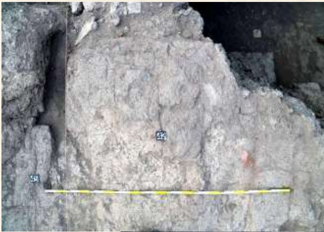
Southern wing of City Gate, US 42
